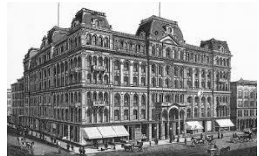
Figure 1.5 Tremont House, Boston
